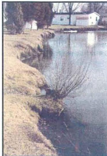
Figure 2: A dramatic example of how woody vegetation will hold soil together, while the adjacent grass cover around this pond has allowed the banks to completely fail, thereby adding to the state's largest water quality pollutant of concern - soil erosion and sedimentation.
