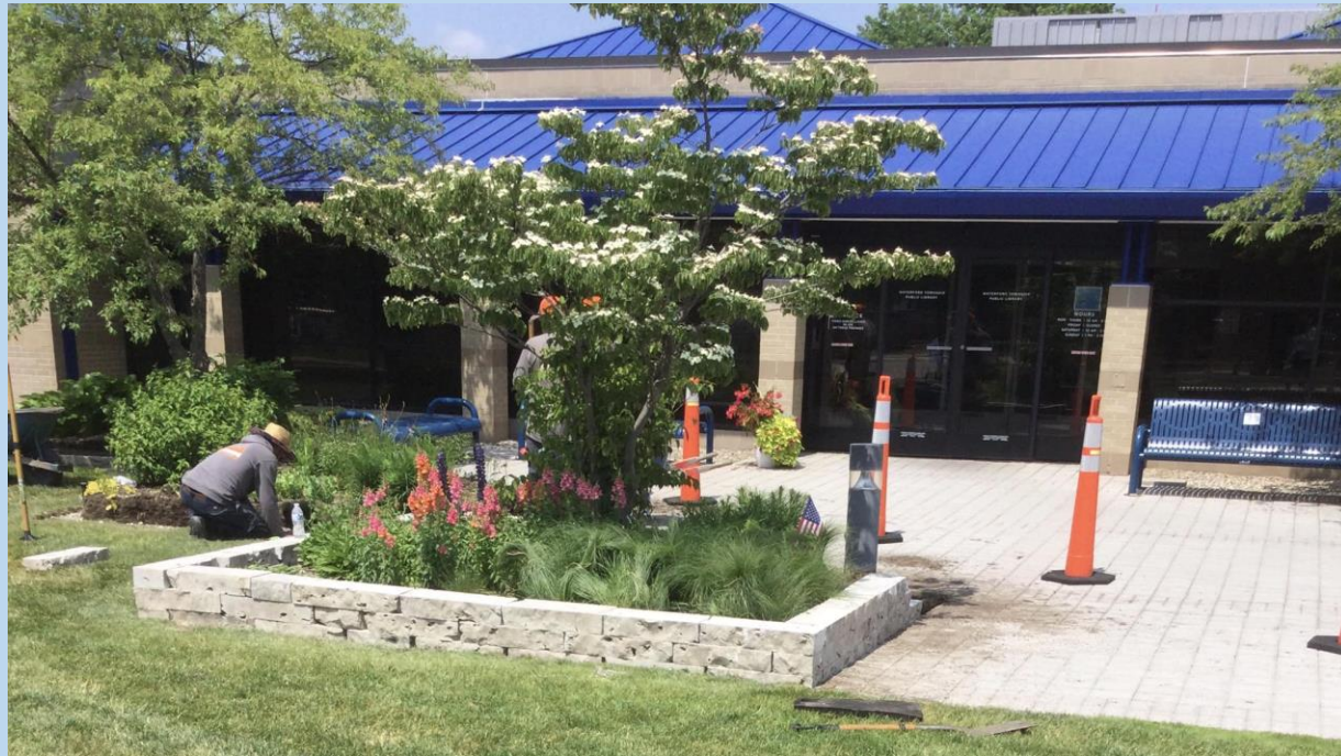
Timber walls replaced with blocks on garden beds
