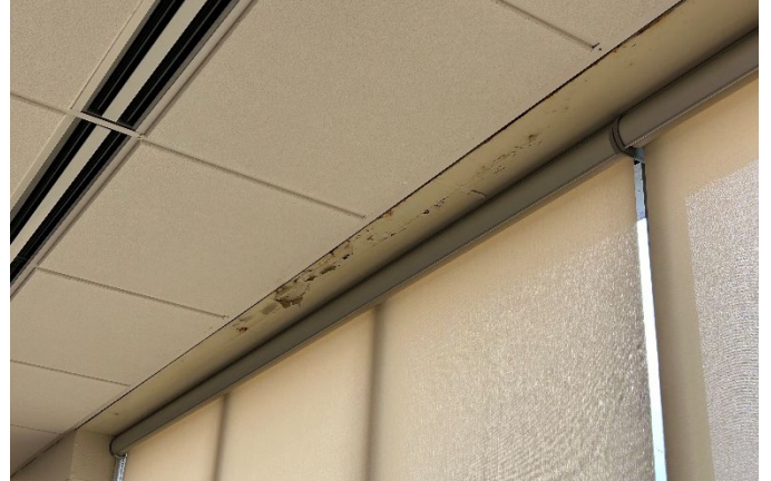
Water Infiltration at Southeast Classroom
