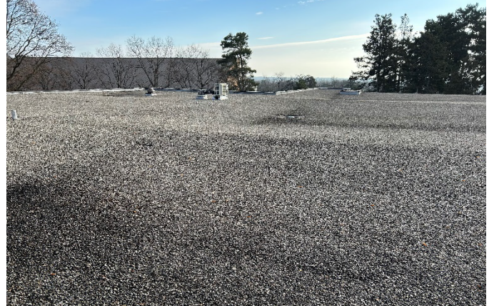
Ballasted Built Up Roof
