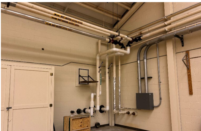
Heating Piping Inlets - NW Corner of Gym
