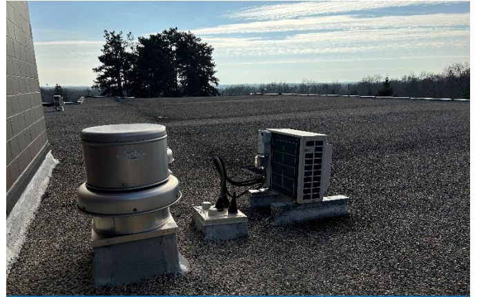
Roof Top Exhaust Fan and A/C Condenser
