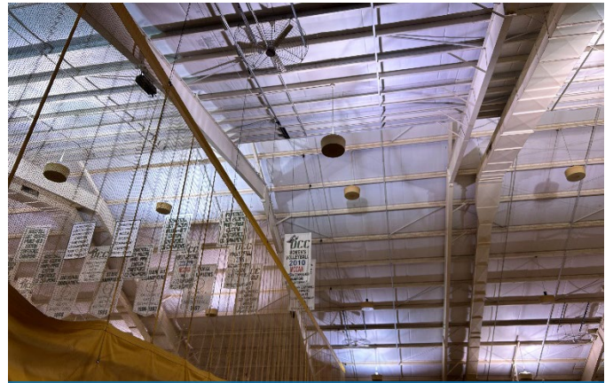
Ceiling Hung Indirect Lighting
