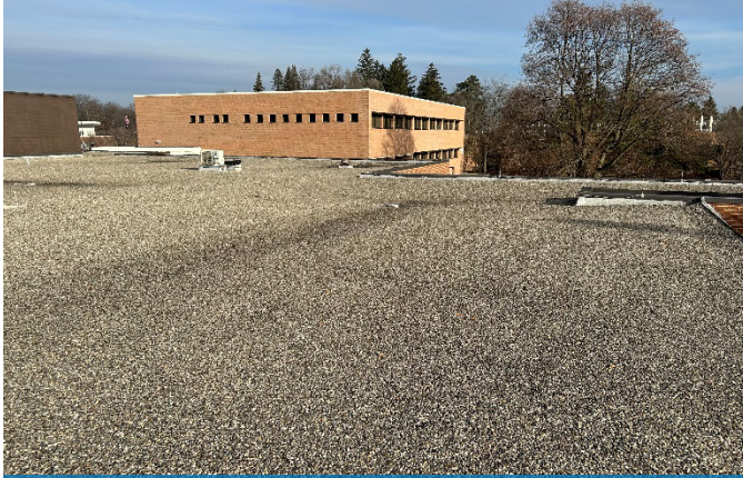
Ballasted Built Up Roof
