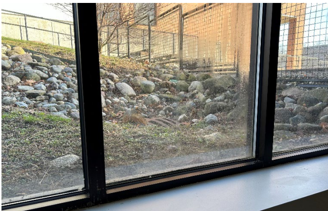
Northeast Window – Broken Seal
