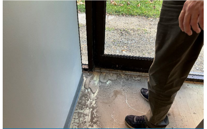
Water Infiltration at East door
