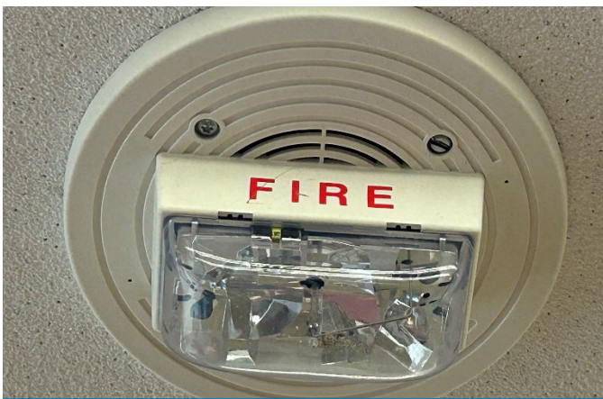
Ceiling Mounted Strobe/Alarm
