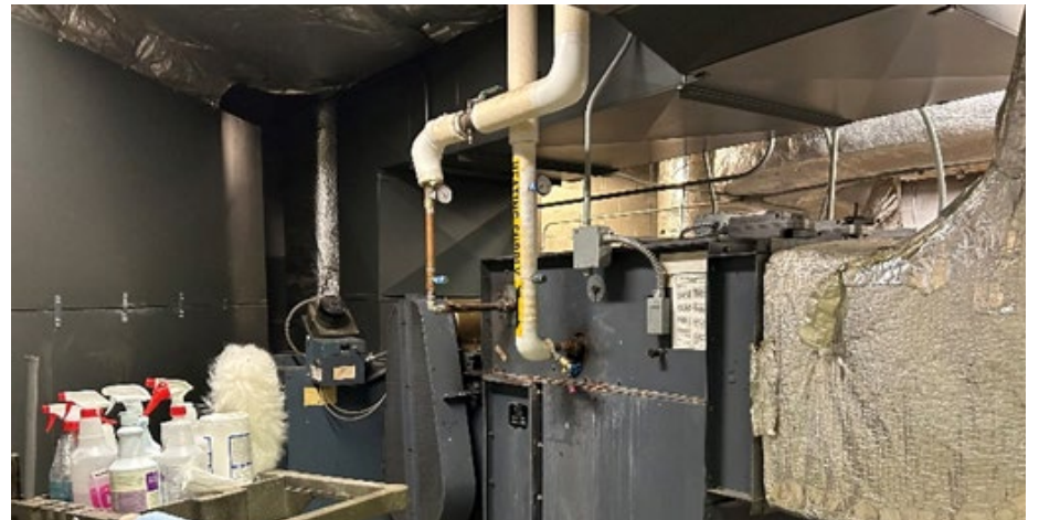
Mechanical room AHU
