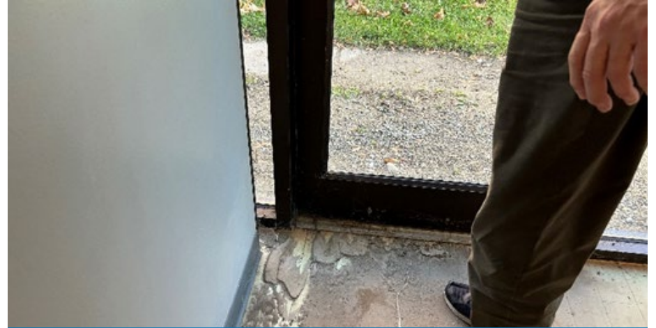
Water infiltration at east door
