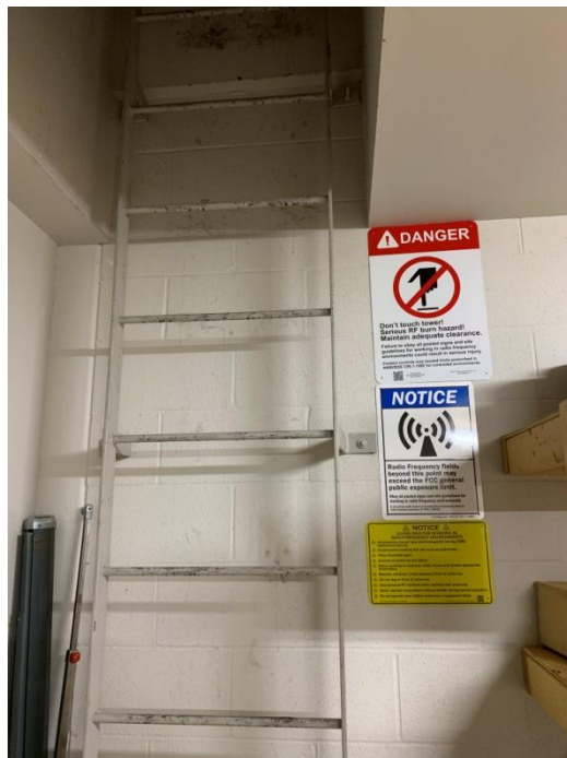
Newly installed radio safety signage at a fire station. This is located at a roof access, warning of transmitting antennas.
