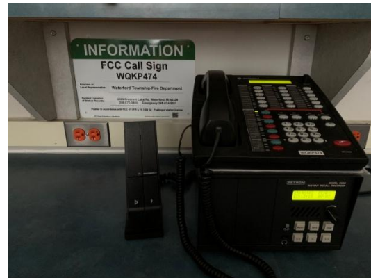
Backup dispatch console at station 1 with tone encoder and instant recall recorder.
