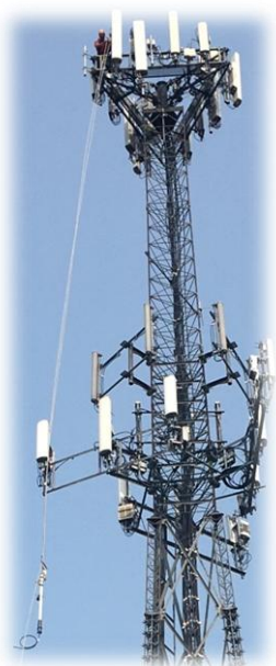
New VHF antenna being hoisted by tower climbers.
