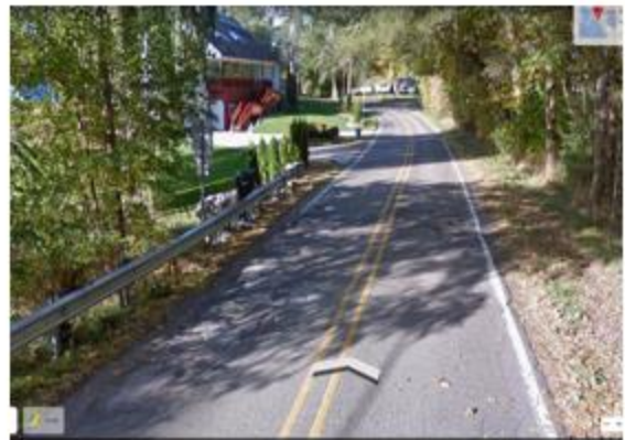
Mann Road (looking westerly near box culvert crossing)
