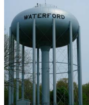
Cass Lake Elevated Water Storage Tank
