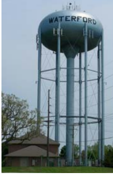
Main Street Elevated Water Storage Tank
