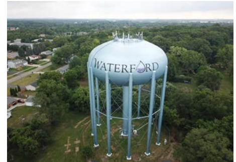
The Cass Lake Road elevated water storage tank stores 1.5 million gallons of potable water.
