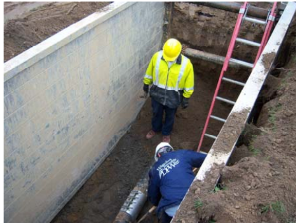
DPW Distribution Branch employees repairing a water main. The Township has 360 miles of water main of various age and composition.
