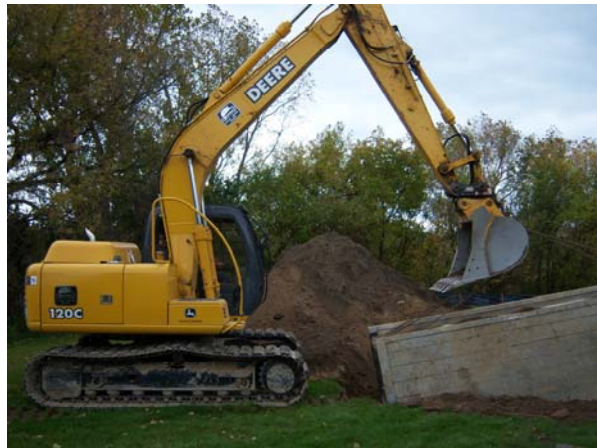
DPW Distribution Branch crew placing a 'Trench Box' in place prior to a water main repair. Trench boxes are used as a safety measure to prevent cave-ins when working near unstable or non reliable soil conditions.
