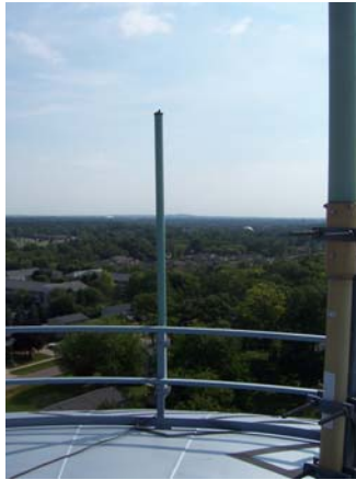
Neptune Omni-Directional Antenna Operating at 450 MHZ located on the Cass Water Tank.
