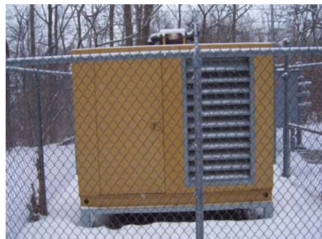
Stationary power generator at one of the Township's 62 sewer pumping stations. At these sites, the generators automatically start and transfer load for continued operation during power failures.
