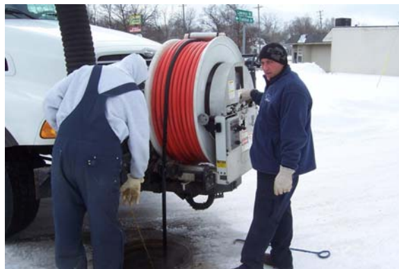
DPW Sewer Branch Employees Jim Cassidy (left) and Scott McGrady (right) working with one of the DPW's two sewer vacor trucks. These trucks and crews are responsible for cleaning 360 miles of Sanitary Sewer within the Township.
