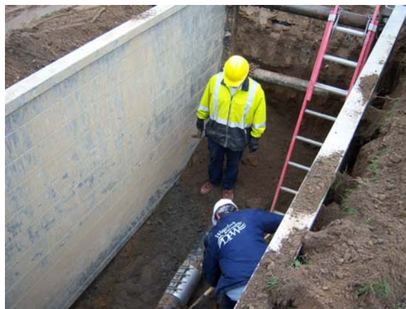
DPW Distribution Branch Employees repairing a water main. Waterford Township has 360 miles of water main of various age and composition.
