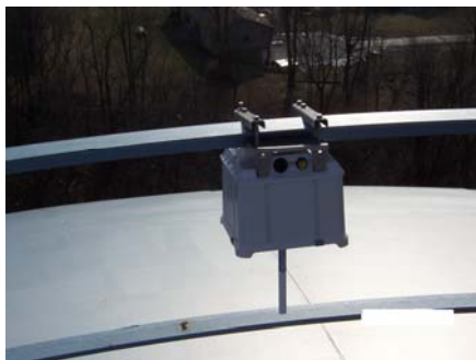
Itron 1.4 GHz Fixed Network Meter Reading Collector Cass Water Tank Waterford Twp. MI
