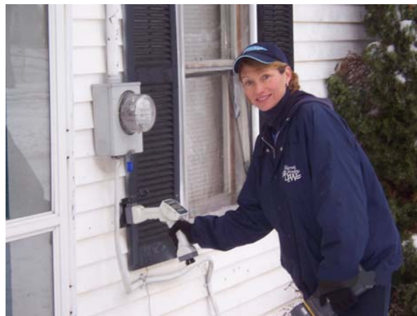
DPW Employee Julie Griffin reading a conventional Meter Reading Interface Unit. The Handheld Device is later Downloaded and Interfaced the DPW's Meter Reading and Billing Software
