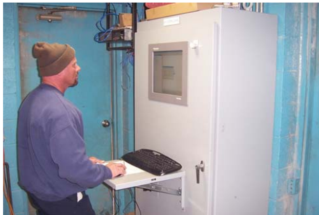
DPW Electrical Branch Employee Jeff Mohr utilizing the Zycom Computer Interface Unit at a Water Treatment Plant. Electrical Branch Employees work extensively with the monitoring systems at the Township's water and sewer sites.
