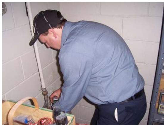
DPW Employee Bill Collier installing a water meter. The water meter has a set of wires connected to an outside meter reading device.
