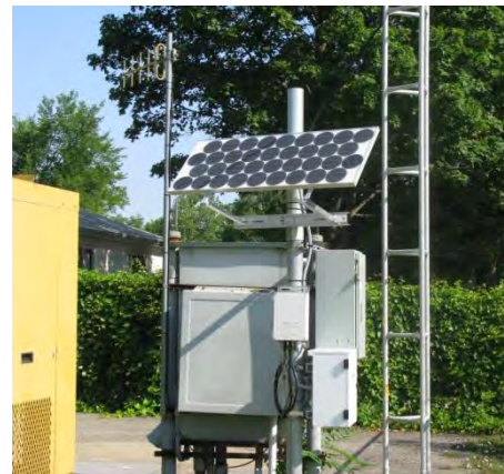
Neptune R-450 Fixed Network Collector site with a solar panel for energy conservation.
