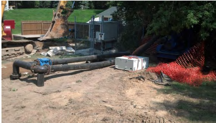
Bypass pumping system in place while work is being completed on the McCormick Dr. sewage pumping station.
