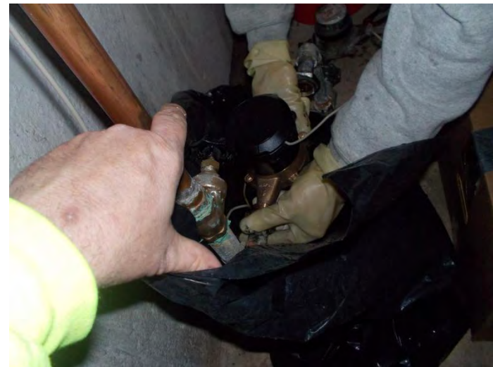
A new water meter is installed
