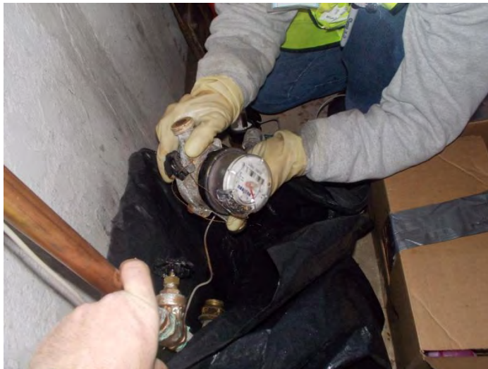
An old water meter is removed from service
