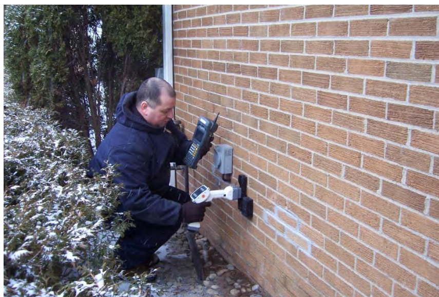
Service Branch employee Dale Dorrance utilizing the DPW's Electronic Meter Reading Equipment to Debug and Troubleshoot a water account. The DPW strives for a high percentage of actual meter reads which reduces the need for estimated utility bills.
