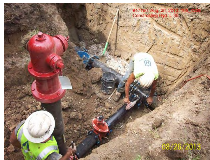
Fire hydrants on any rehabilitated mains were replaced
