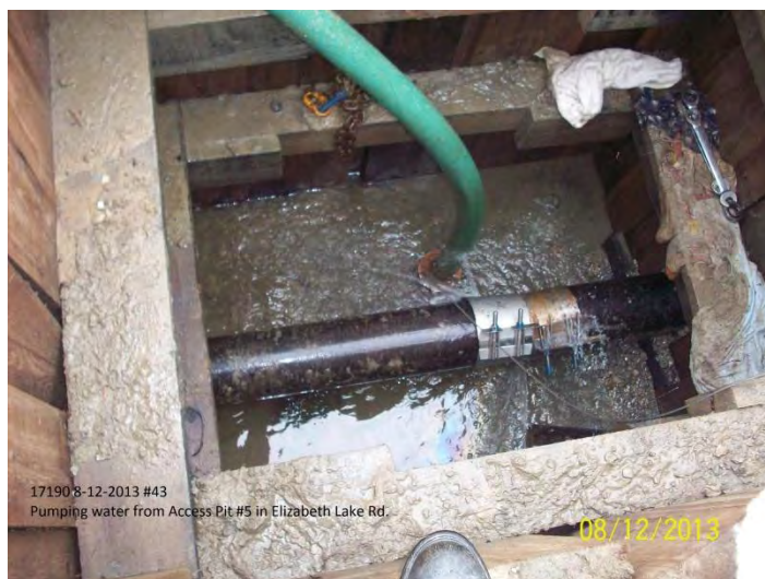
Access pit undergoing dewatering
