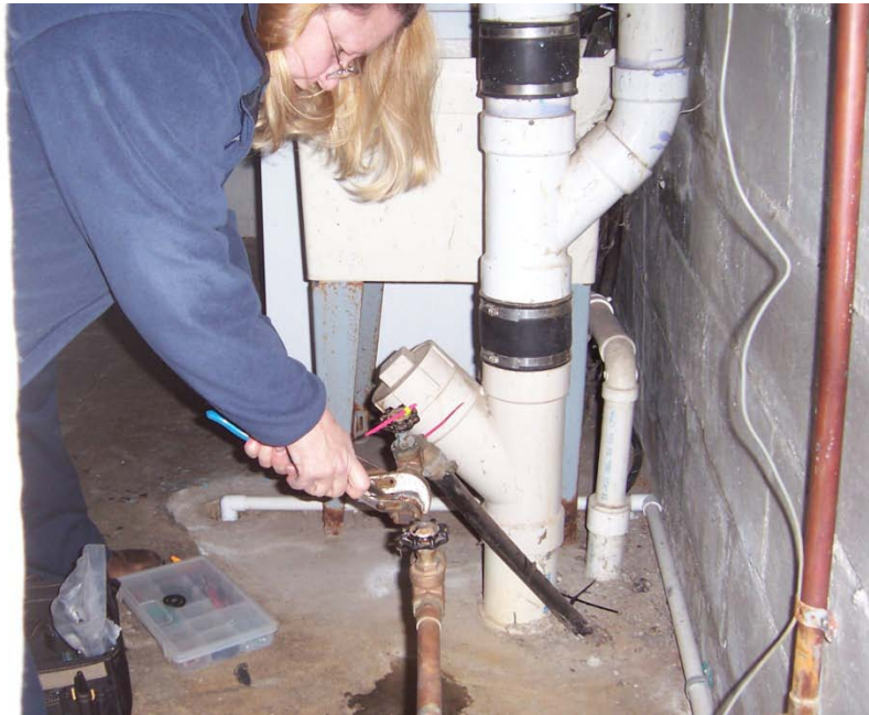
Service Branch employee Dawn Zormeier installing a water meter. The water meter has a set of wires connected to an outside reading device. New meters monitor and alarm on leak detection, reverse flow and no flow. In addition, meter reads are transmitted to fixed collectors that are connected to the Township's Broadband Wireless Network which sends the reads directly to the DPW Office for processing.
