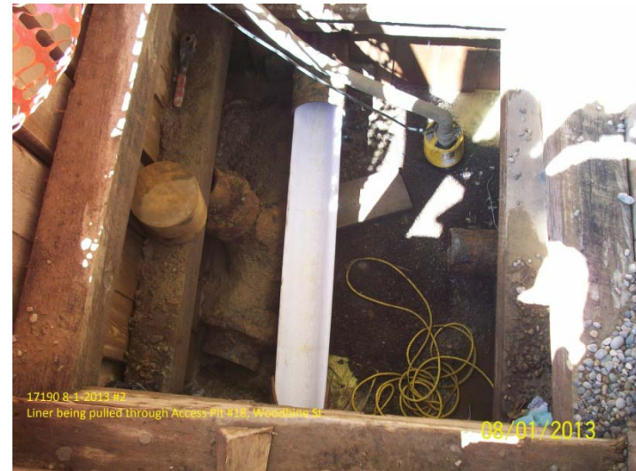
Cured-in-place water main liner is pulled into existing aging water mains.
