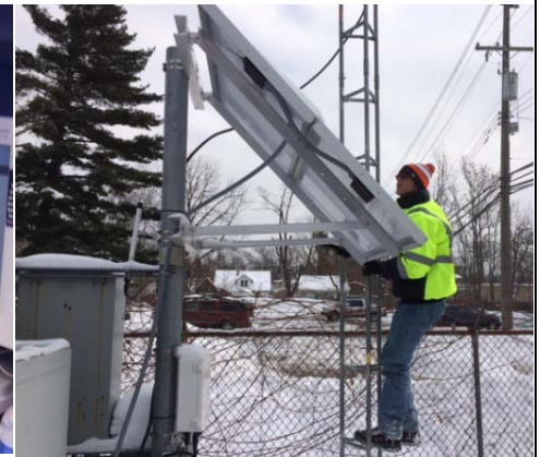
Jim Yearsin of Neptune Technology adjusting the Solar Panel that powers one of Waterford's Fixed Network Collector Sites.
