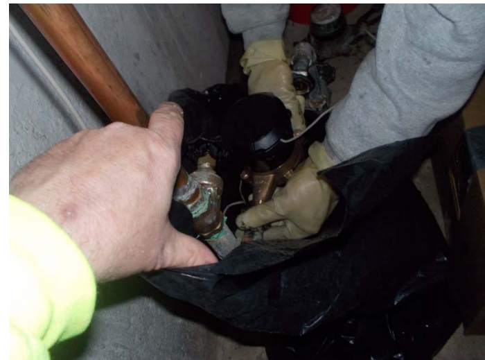
A new water meter is installed
