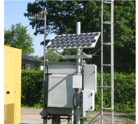
Neptune R-450 Fixed Network Collector site with a solar panel for energy conservation.
