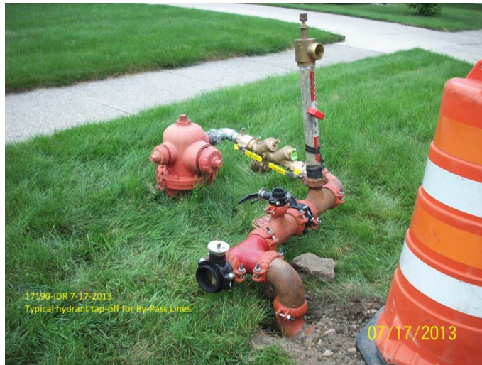
Temporary water services is established and provided through specialized fire hydrant taps.
