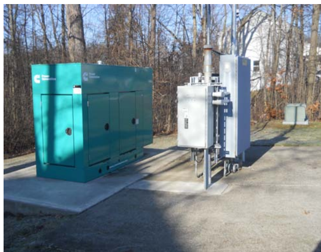
Natural gas generators similar to the ones located at 5477 Lockwood and 3320 Gilchrist Ct. lift stations were purchased with the help of the RAP Grant program offered by MMRMA
