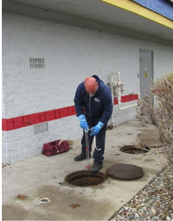
DPW employee Brandon Sluiter conducting an inspection on a grease interceptor at a local facility within the Township
