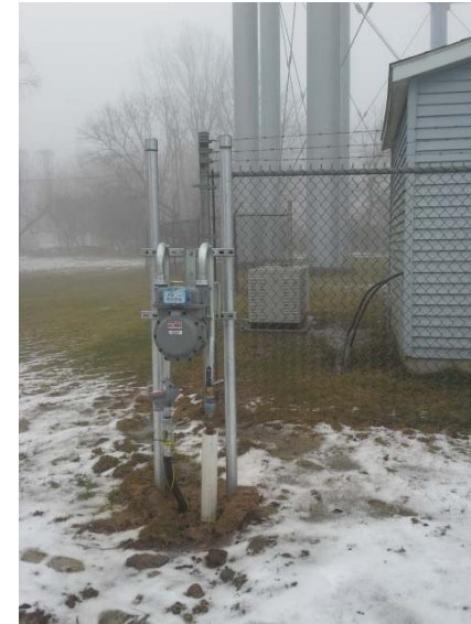
Utility meter for natural gas generator
