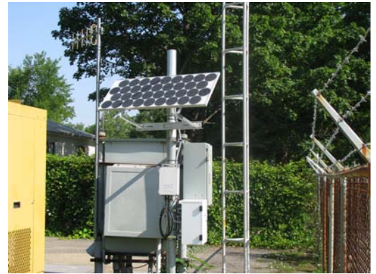
Neptune R-450 Fixed Network Collector site with a solar panel for energy conservation.
