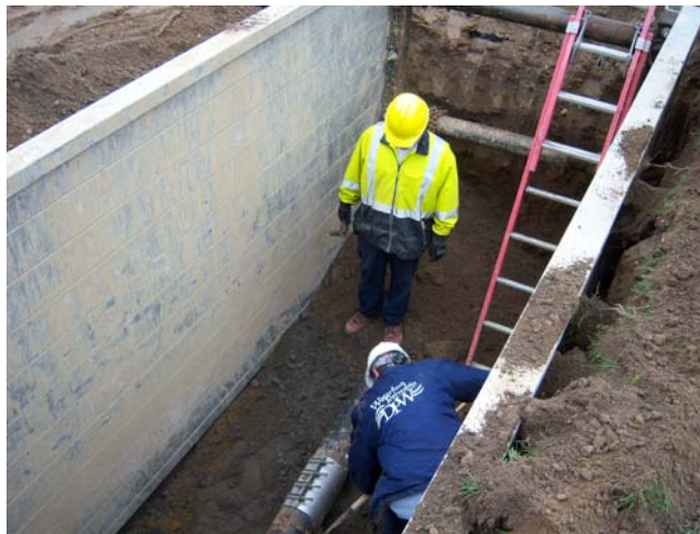
Distribution Branch employees repairing a water main. The Township has approximately 360 miles of water main of various age and composition.
