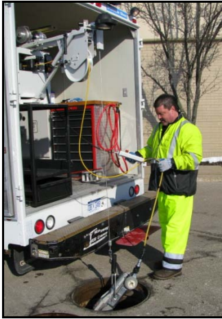
Joe Ashley Lowering CCTV Camera into Sewer Manhole
