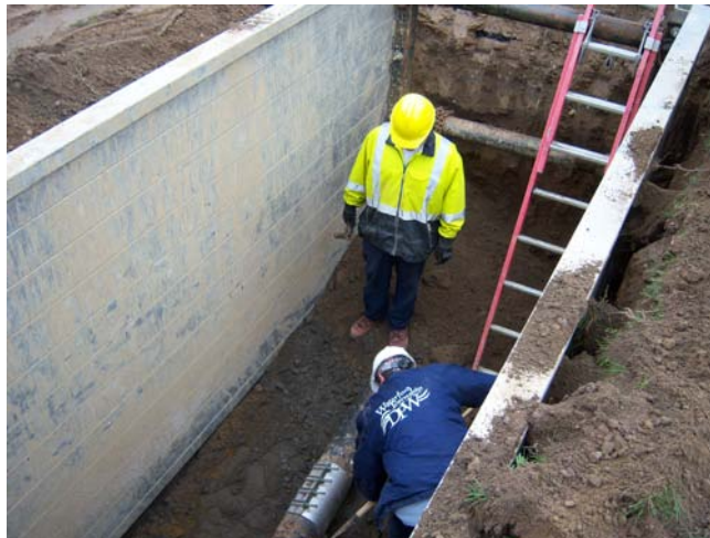
Distribution Branch employees repairing a water main. The Township has 360 miles of water main of various age and composition.
