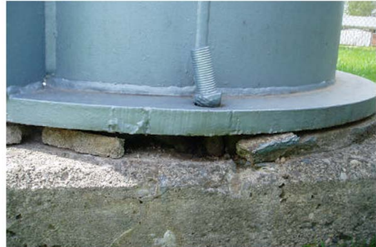
Leg shifted with bent anchor bolt and broken grout.
