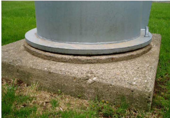
Leg of Tank showing shift towards center and large gap between leg and baseplate grout.
