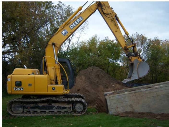
Distribution Branch crew placing a 'Trench Box' in place prior to a water main repair. Trench boxes are used as a safety measure to prevent cave-ins when working near unstable or non reliable soil conditions.
