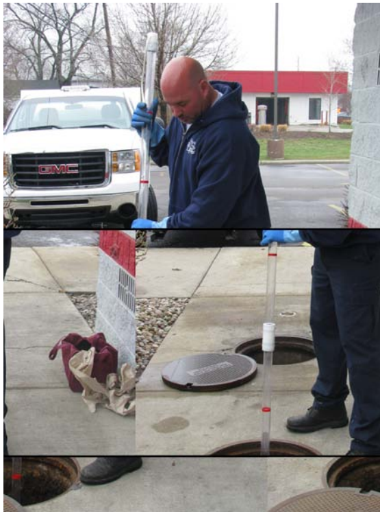
DPW employee Brandon Sluiter conducting an inspection on a grease interceptor at a local facility within the Township
