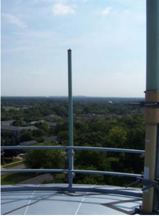
Neptune Directional Antenna Operating at 450 MHZ located on the Cass Water Tank.
