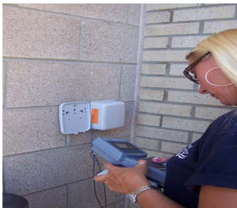
Service Branch employee Penny Holden configuring R-450 Reading Devices in the Field.
