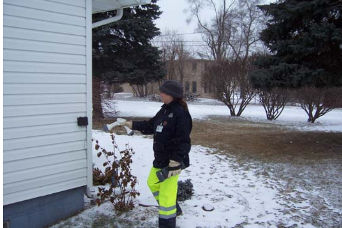
Service Branch employee Heather Krupic reading a conventional Meter Reading Interface Unit. The Handheld Device is later downloaded and interfaced with the DPW's Meter Reading and Billing Software Systems.
