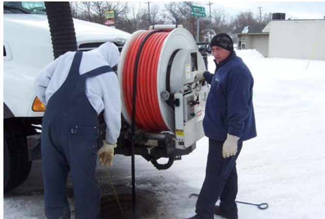
DPW Sewer Branch employees, Jim Cassidy (left) and Scott McGrady (right), working with one of the DPW's two sewer vactor trucks.
