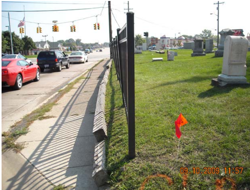
The picture above depicts the slanted and eroded wall slope prior to repair.
