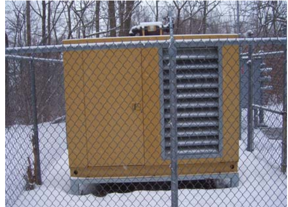
Stationary power generator at one of the Township's 62 sewer pumping stations. At these sites, the generators automatically start and transfer load for continued operation during power failures.
