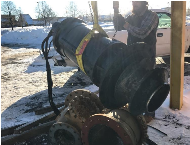
Crews remove an old pump
