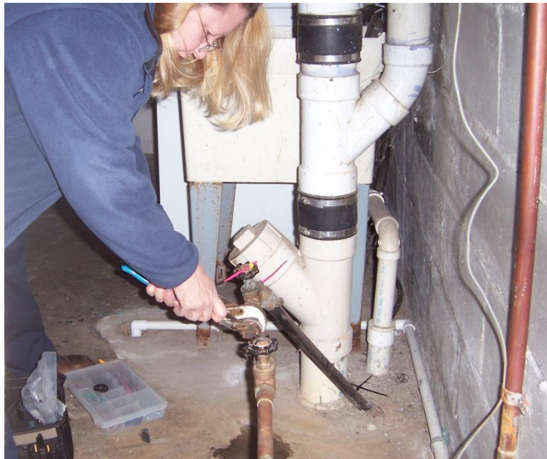
Service Branch Foreman Dawn Zormeier installing a water meter.
