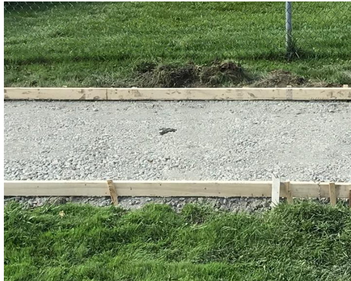
A section of sidewalk being laid out and formed up for repair in 2016.
