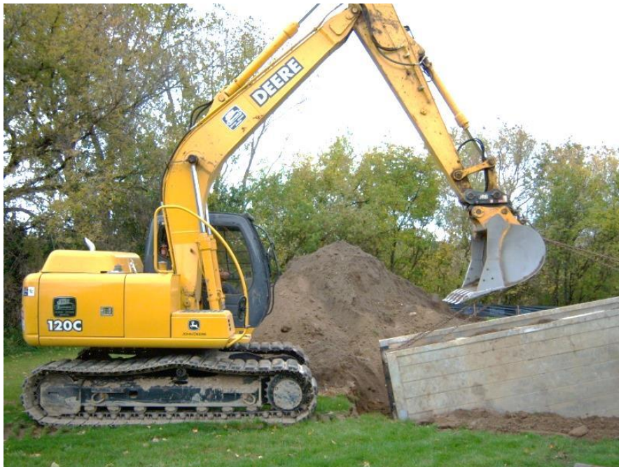
Distribution Branch crew placing a 'Trench Box' in place prior to a water main repair. Trench boxes are used as a safety measure to prevent cave-ins when working near unstable soil conditions.
