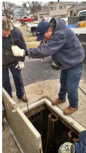
DPW Sewer Branch employees, Walter Reed (left) and Randy Bunce (right), pulling a pump at one of Waterford's 62 sewer lift stations.
