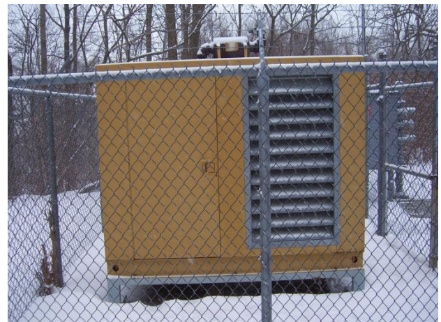
Stationary generator at one of the Township's 62 sewer pumping stations. At these sites, the generators automatically start and transfer load for continued operation during power failures.
