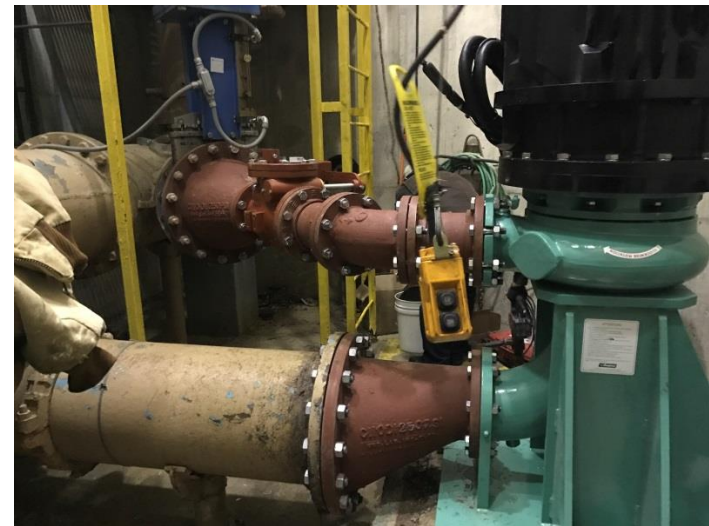
Newly installed pump and piping
