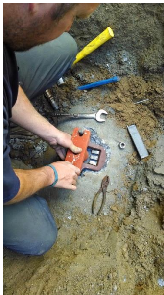
Distribution Branch Employee Frank Patrello conducting a water tap on a 20" steel reinforced watermain.
