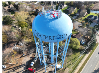
The elevated water storage tank at Main Street and Walton Blvd. stores 0.75 million gallons of potable water
