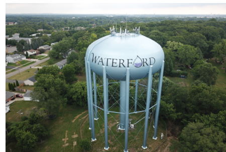
The elevated water storage tank on Cass Lake Road stores 1.5 million gallons of potable water
